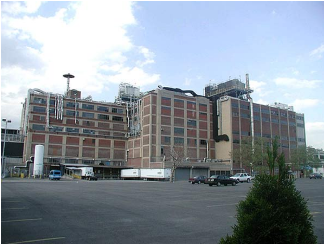
Figure 3: The Former Pfizer Building
